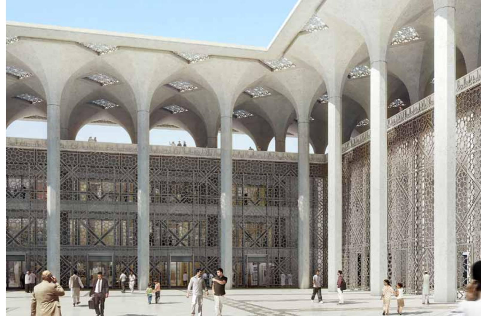
The esplanade with 22-meter high rows of columns
