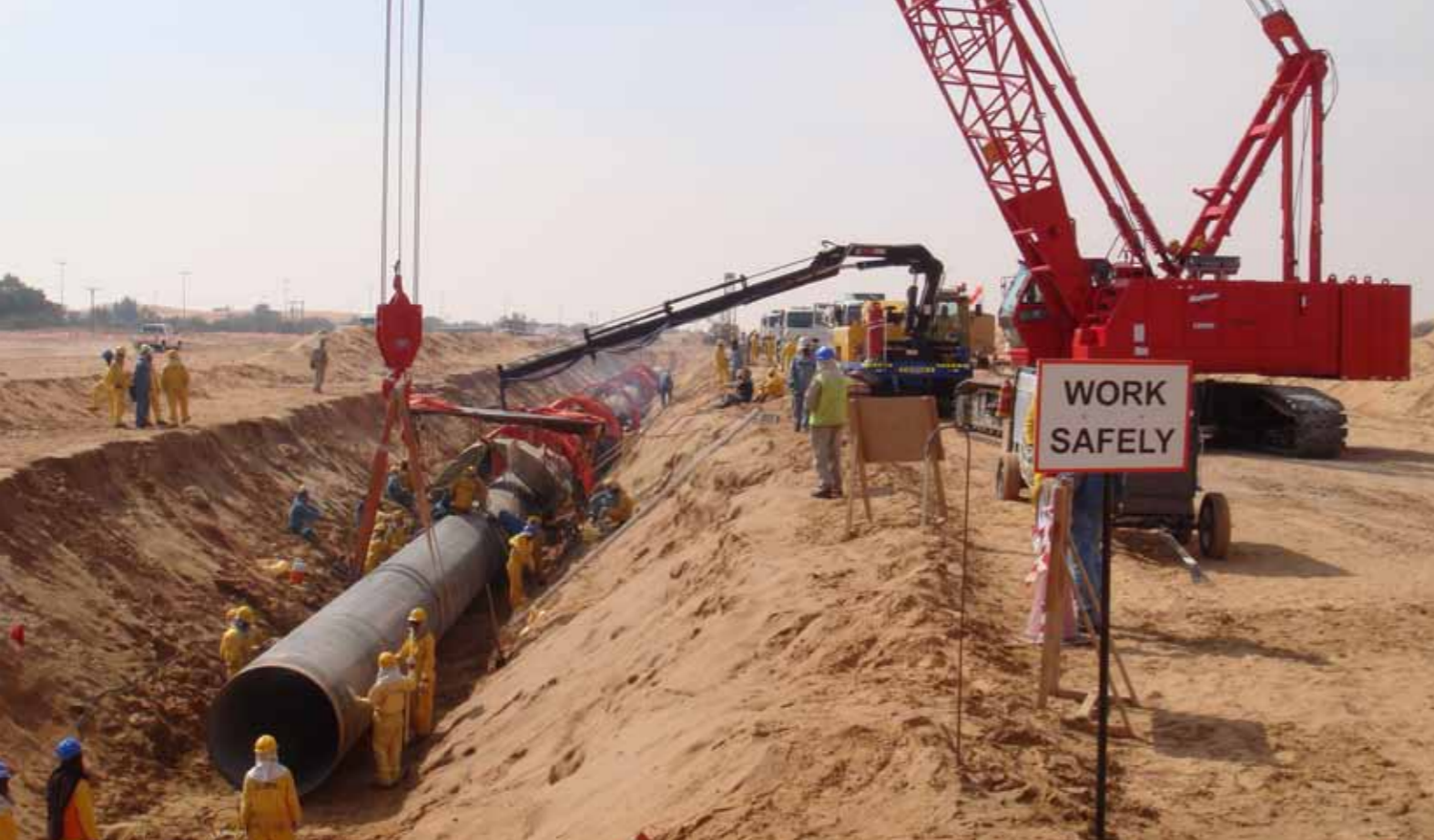
Middle East pipeline installation
